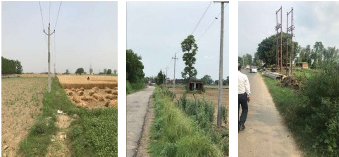
Photo 2: Feeder Separation Works
