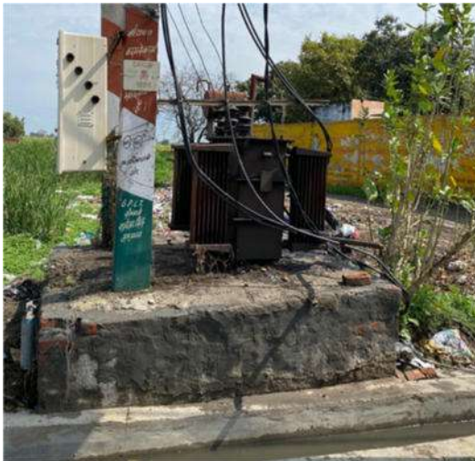
Photo 7 and Photo 8: Poor Installations Posing Community Health and Safety Risk
