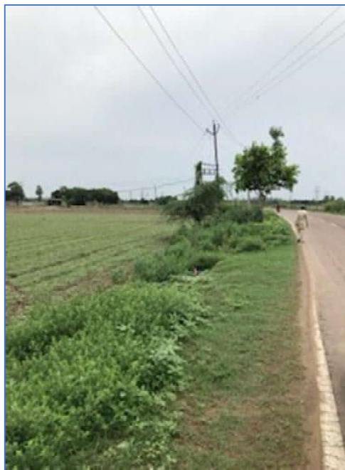
11 kV line along existing road RoW
