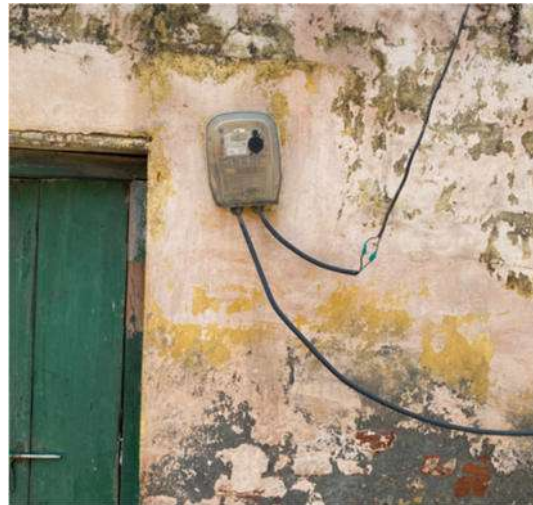
Photo 7 and Photo 8: Poor Installations Posing Community Health and Safety Risk
