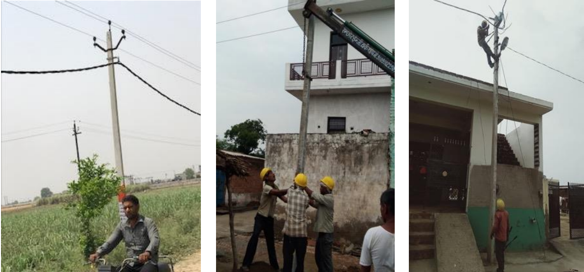
Photo 1: ABC Installation and Stringing Work
