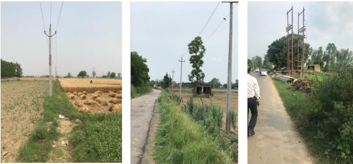
Photo 2: Feeder Separation Works
